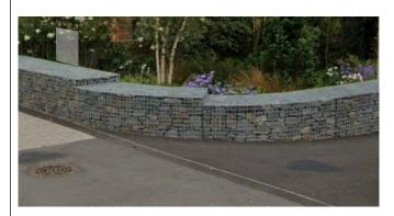
The gabions – essentially steel cages containing stones – link to form a robust wall (see below) but are also capable of having planting incorporated within them. This could take
